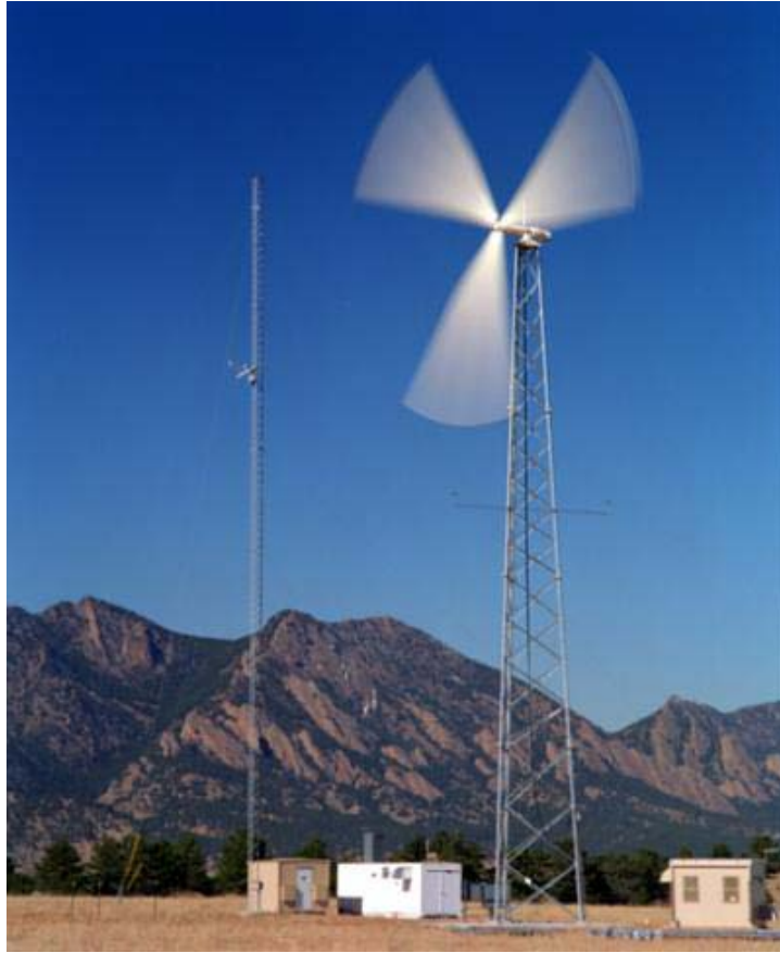
Figure 1. Overall configuration of the AOC 15/50 test turbine.
