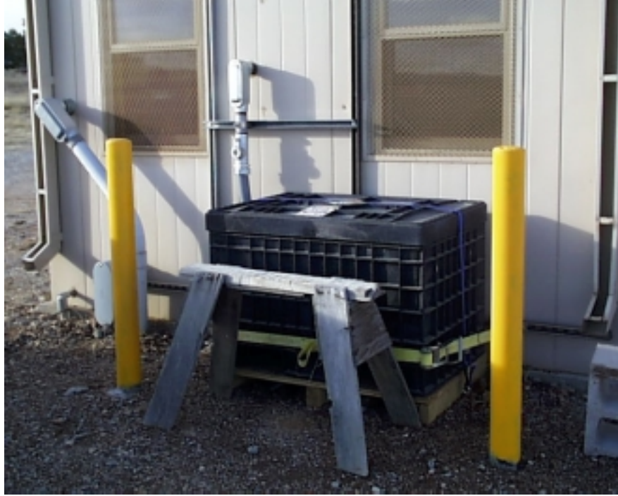
Figure 5. Detail of Battery Box Installation
