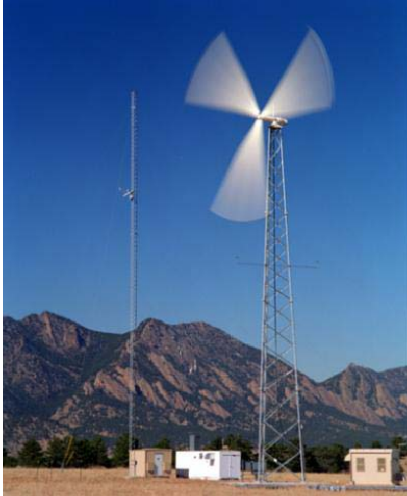
Figure 2. The AOC 15/50 test turbine.
