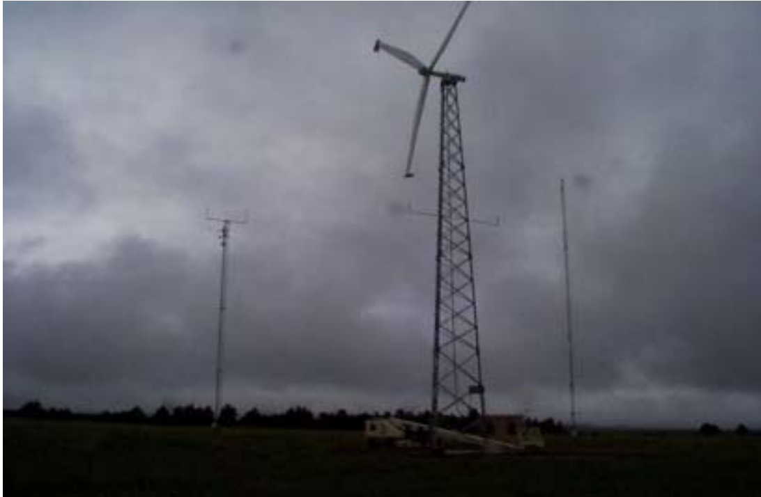
Figure 12. Picture Taken From the Reference Microphone Position (manlift was not present during test)
