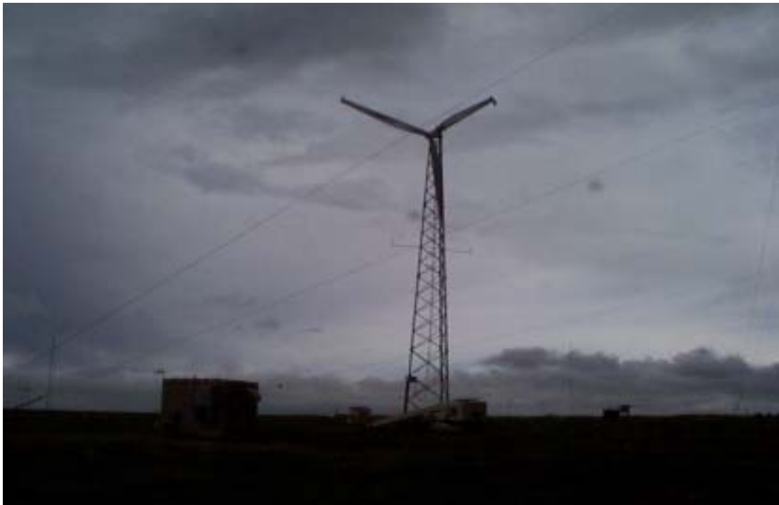
Figure 13. Picture Taken From the Meteorological Tower (manlift was not present during test)
