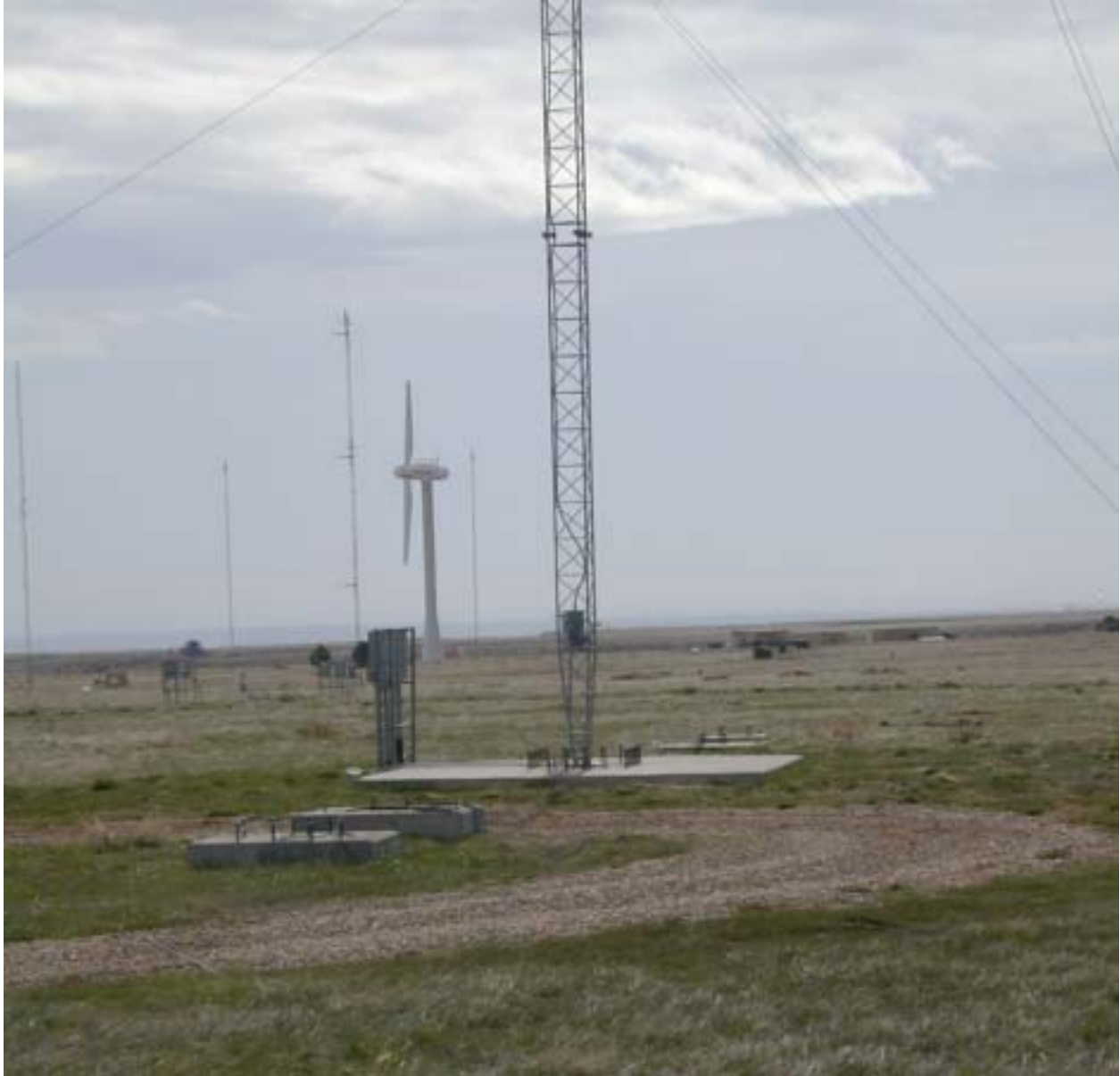
Figure 23. Picture taken from the meteorological tower. (Picture not taken during test.)
