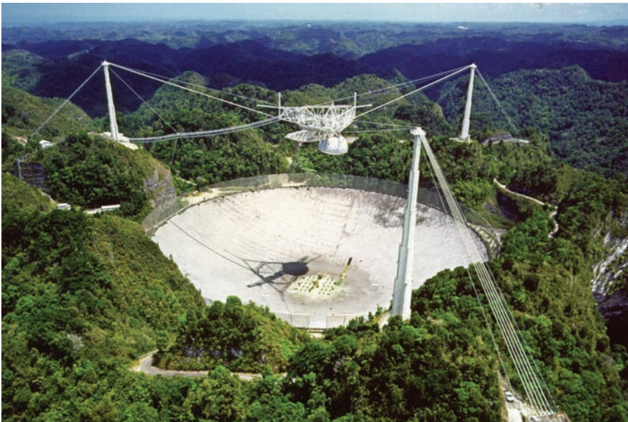
The NAIC facility's 305-meter-diameter reflector is the world's largest single-dish radio telescope. It is used to conduct research in radio astronomy, planetary radar and terrestrial aeronomy.
