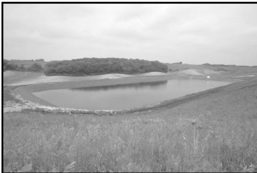
Wastewater Treatment Lagoon Photo courtesy of Clay Smith, Iowa DNR
