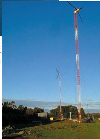
The Isla Tac Power system provides power to the islands' 82 families.
