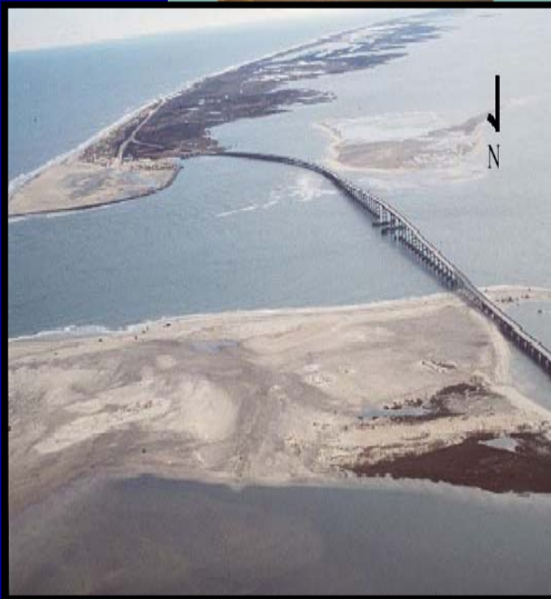
Bonner Bridge, Oregon
