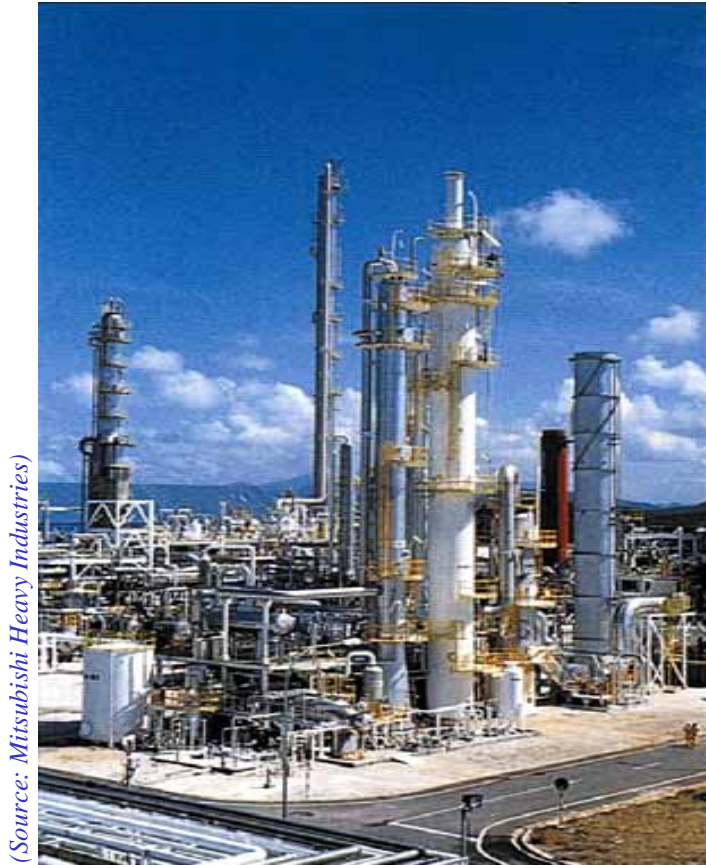
Post-Combustion Capture ( gas-fired power plant, Malaysia )
