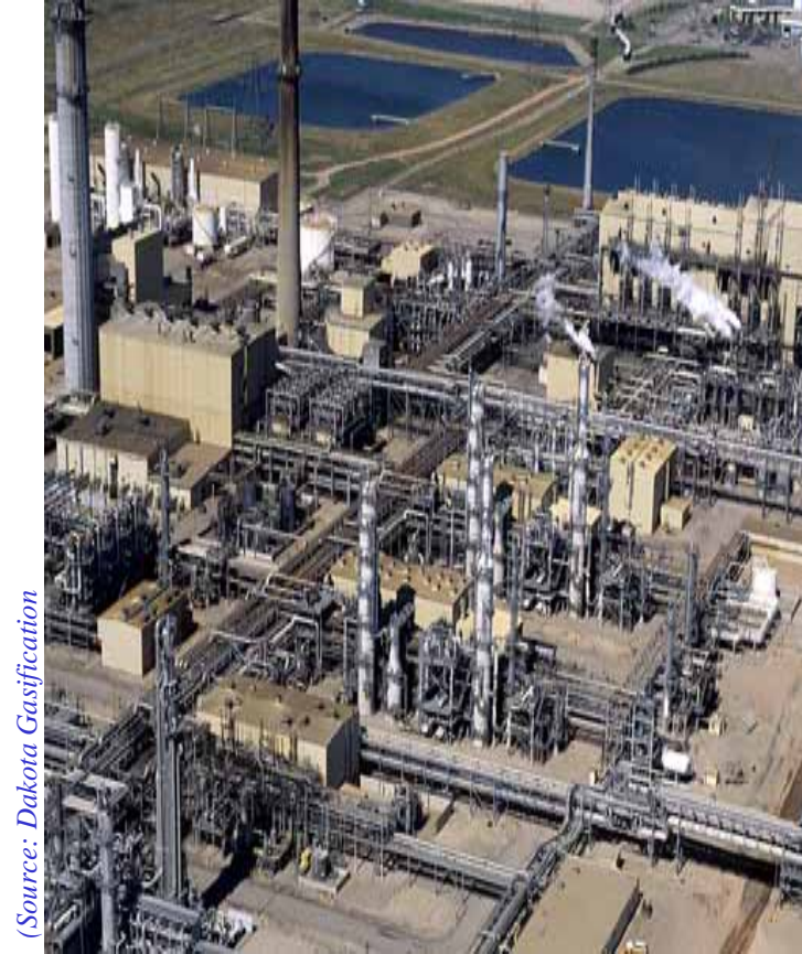
Pre-Combustion Capture ( coal gasification plant, USA )
