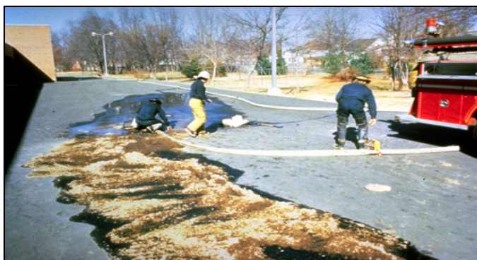
The first responders at the scene of a release of a hazardous substance are usually fireman or state or local police. They conduct the initial assessment of the situation and take emergency actions such as fighting a fire, securing the area, or re-routing traffic.
