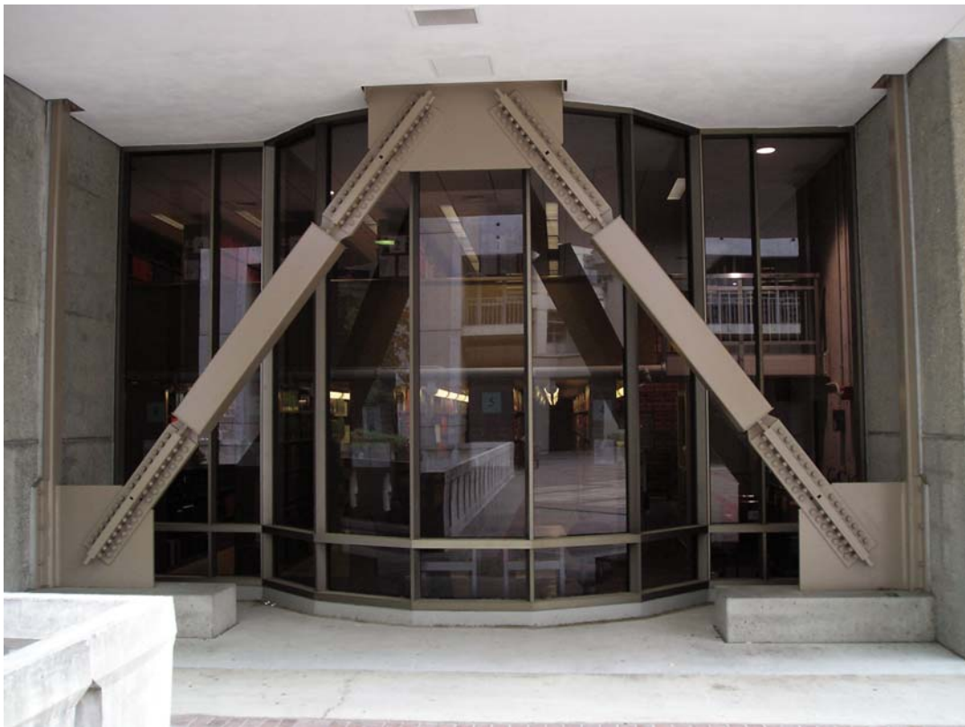
Figure 14. Hildebrand Hall: unbonded braces.
