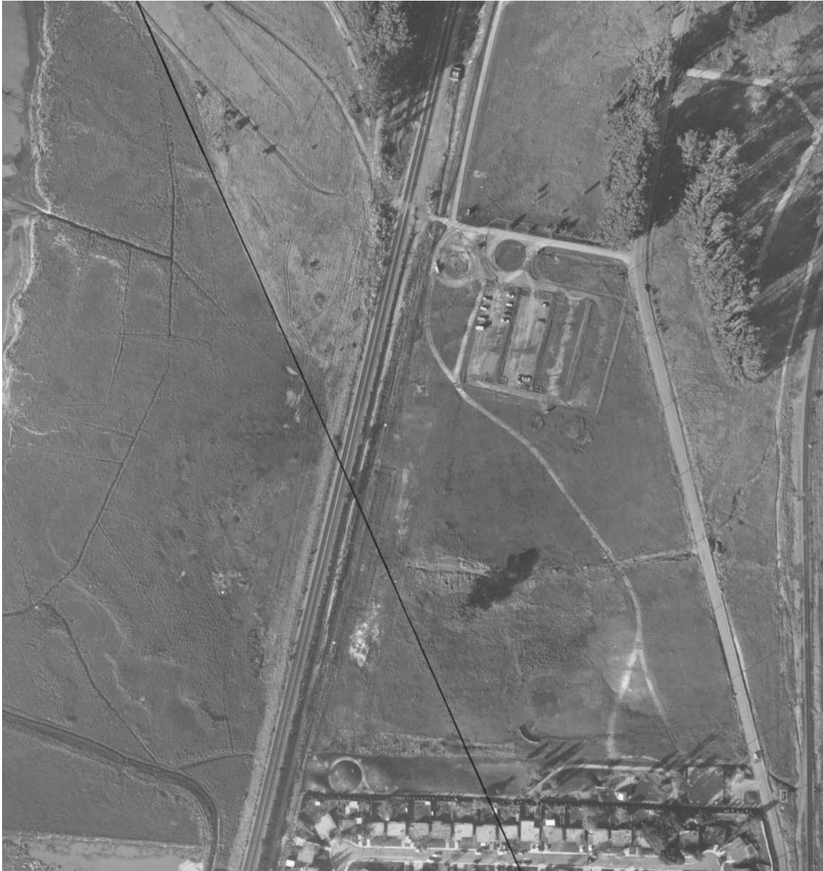
Figure 23. 1978 aerial photo of the Hayward fault as it passes through Parchester Village, offsets two pipelines and the Union Pacific railroad tracks, and then forms the linear scarp along the tidal marsh.
