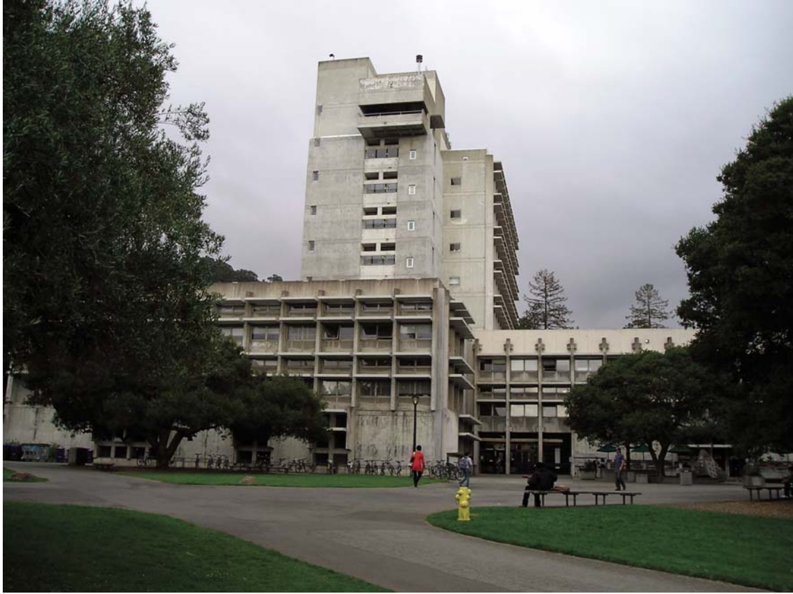
Figure 18. Wurster Hall, western façade.
