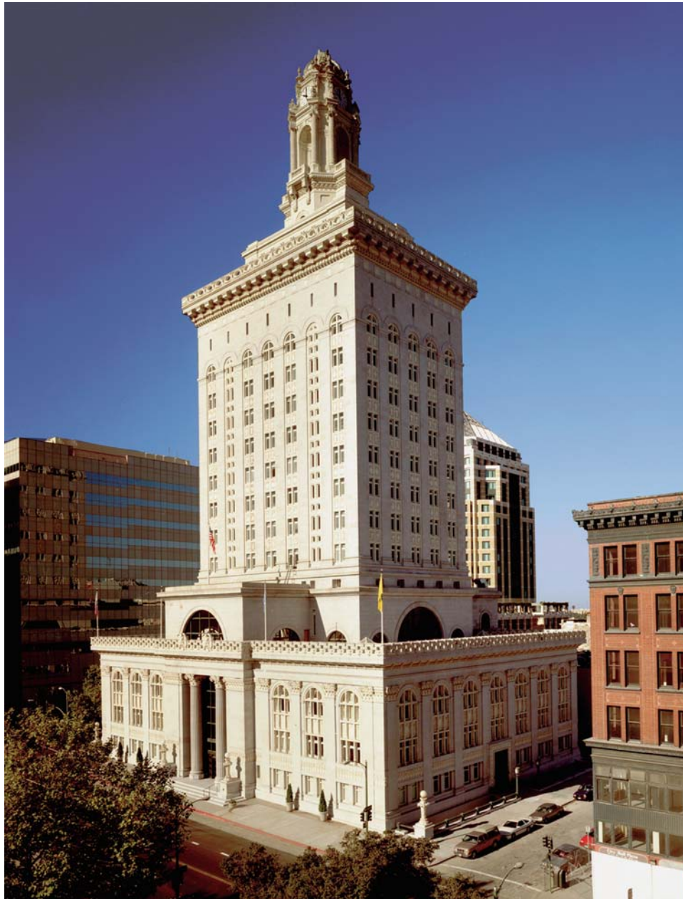
Figure 38. Photograph of Oakland City Hall (from Steiner and Elsesser, 2004).
