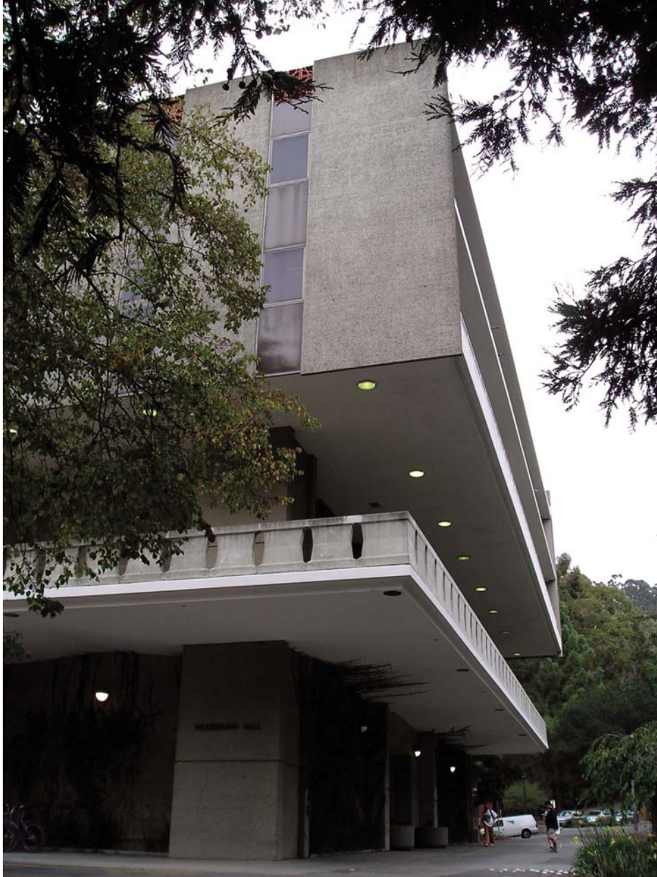
Figure 12. Hildebrand Hall seen from the southwest.
