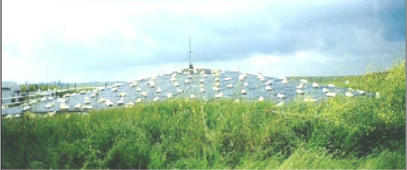
Landfill bioreactor cell, Yolo County, California
