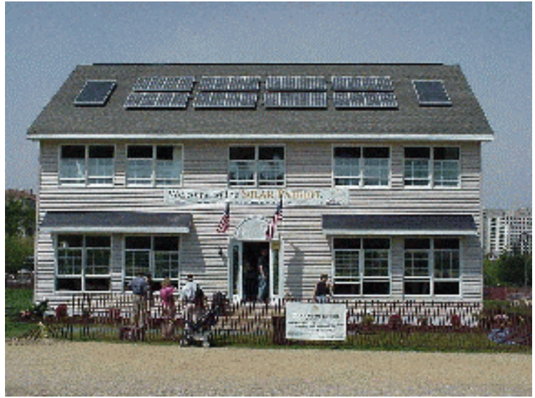
Zero-energy home, the “Solar Patriot.”
