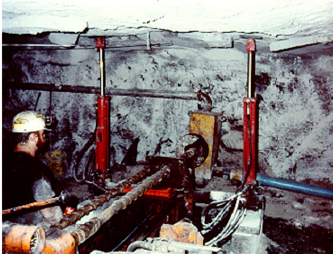
In-mine directional drilling.
