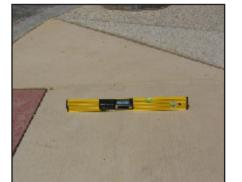
Figure 2: Non-compliant newly installed sidewalk curbcut
