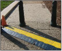
Figure 1: Non-compliant temporary sidewalk ramp
