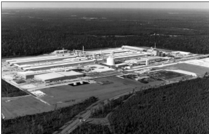
Alumax Mount Holly Aluminum Production Facility
