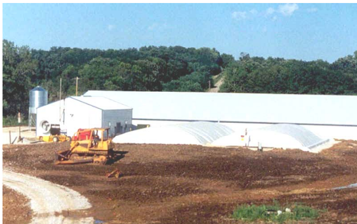
Construction of a complete mix anaerobic digestion system
