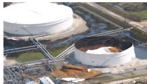
Chevron Empire Terminal tank damage. Photo: Chevron Inc.
