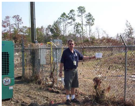
PHMSA Transportation Regulations Specialist Gary McGinnis, on special hurricane survey detail in Lake Shore, Miss., to locate and inspect pumping station damage.
