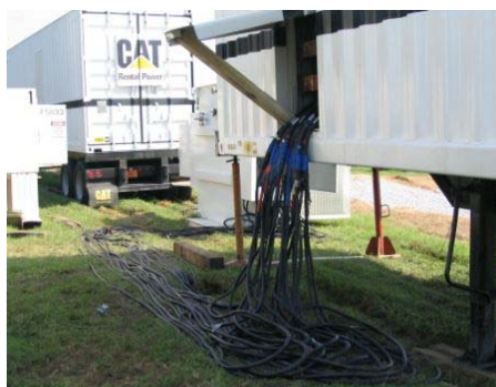
Emergency crews work to connect one of several mega-watt electrical generator trailers to meet the supplemental power requirements needed to restore operations at Colonial Pipeline and Plantation Pipeline pumping stations, storage tanks, and truck loading terminals in Collins, Miss.
