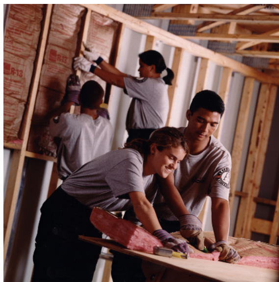
AmeriCorps members building homes with Habitat for Humanity.
