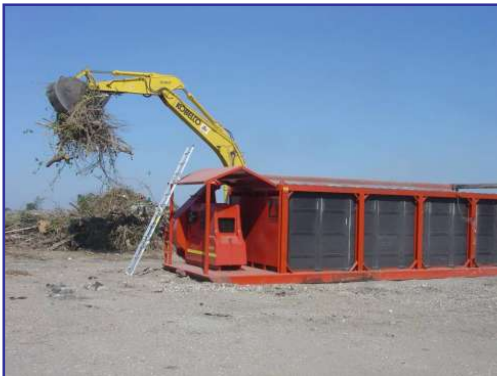
Figure A-5. Particulate emissions during charging of ABT and during vegetative debris handling at Amid Landfill (October, 25, 2005).
