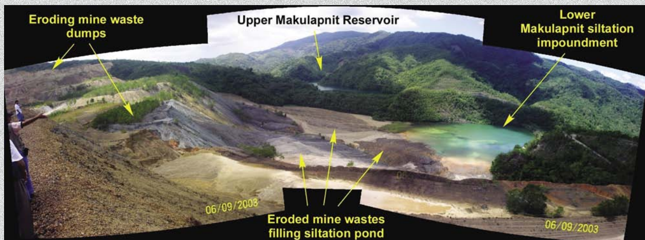
Photographic panorama showing erosion of mine waste dumps into the lower Makulapnit siltation impoundment pond on Marinduque Island, Philippines. Digital composite of three photographs by H. Miller and J. Madsen, taken in June 2003.
