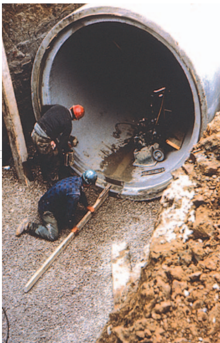
Workers install sewer line
