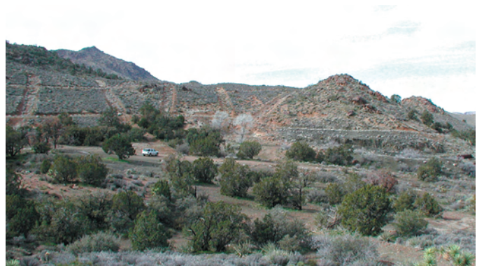
Figure 11. View of trenches and a small open-cut pit at the Gold Butte Vermiculite Mine (the western wall of the pit is in the right middle ground at the base of the hill). The vehicle is parked at the approximate site of the old vermiculite mill.
