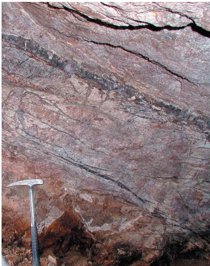
Figure 39. Shallowly northwest-dipping sheared, altered, and silicified gold-bearing zone (behind hammer) in an adit at the Silver Bell Mine. Site of samples AP-015 and AP-015C.
