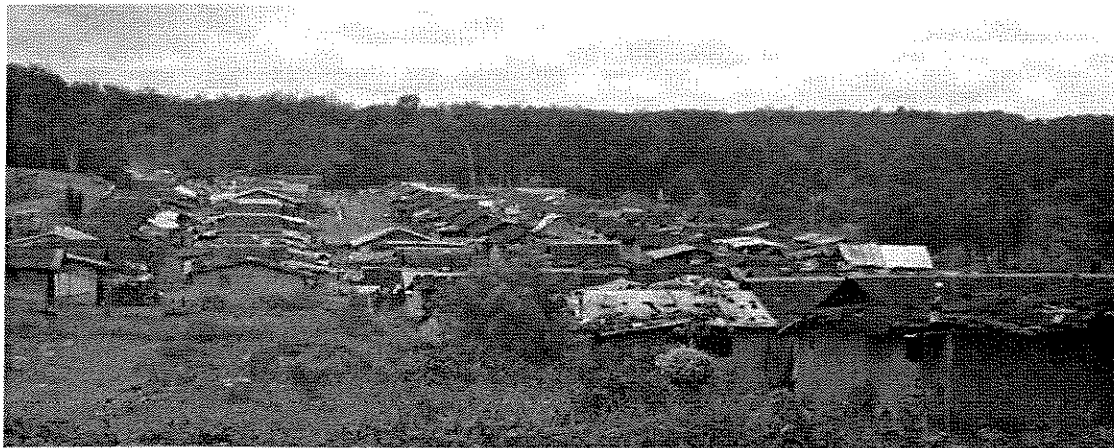
Division 41, photo taken by HRO on visit of 25 July, 2005. started renovations in 1990 but stopped due to the war. Renovations in three camps began in 2005.
