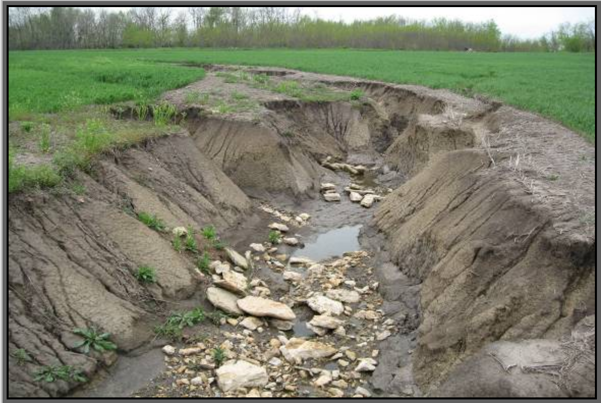
The 150 Highway & Botts Road PIEA Planning Area – Resolving Topographic Issues
