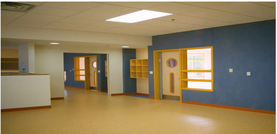
Child-scaled windows in the wall and doors in childcare center in Kansas City, MO
