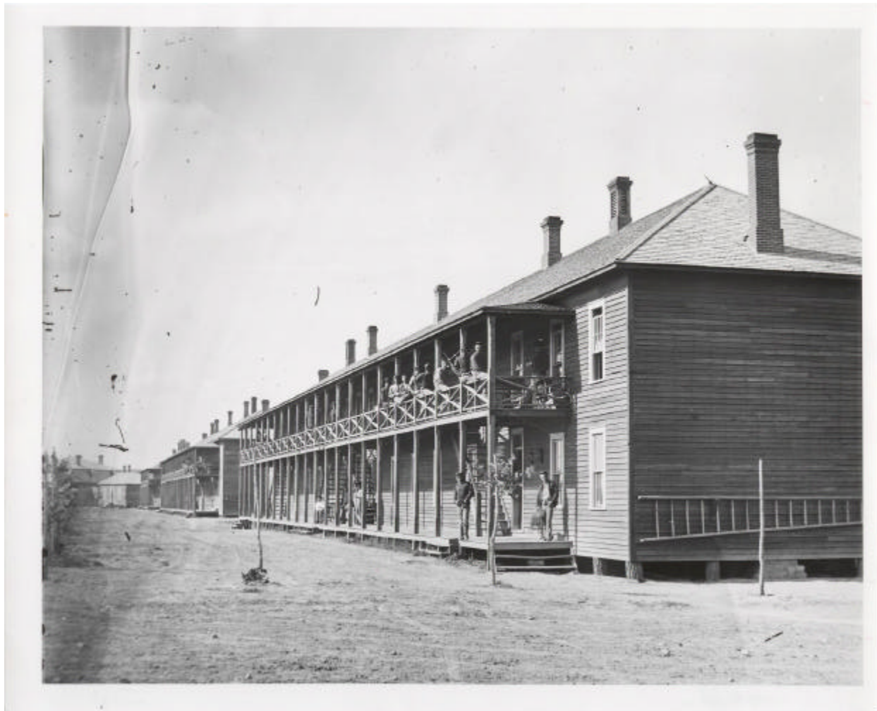
Figure 5. Cavalry barracks in 1880. The following year the second barracks back was destroyed by fire and replaced with a single story brick structure used as the guardhouse. The troopers shown are most likely from the Second Cavalry. (Courtesy of Coffrin's Old West Gallery.)
