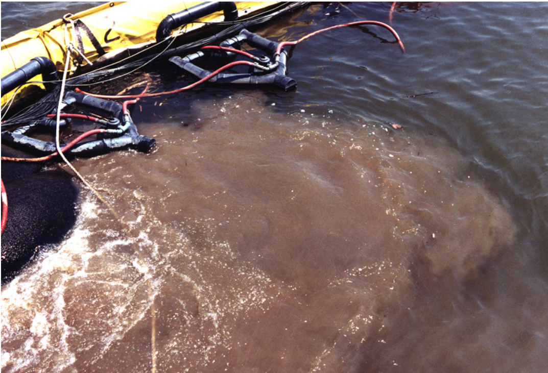
Photo 2. Lovett 1998 Gunderboom® MLES™ Deployment with AirBurst™ Technology at the Lovett Generating Station, Tomkins Cove, NY.
