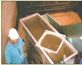
Temporary Latent Impingement Mortality (LIM) Holding Tank
