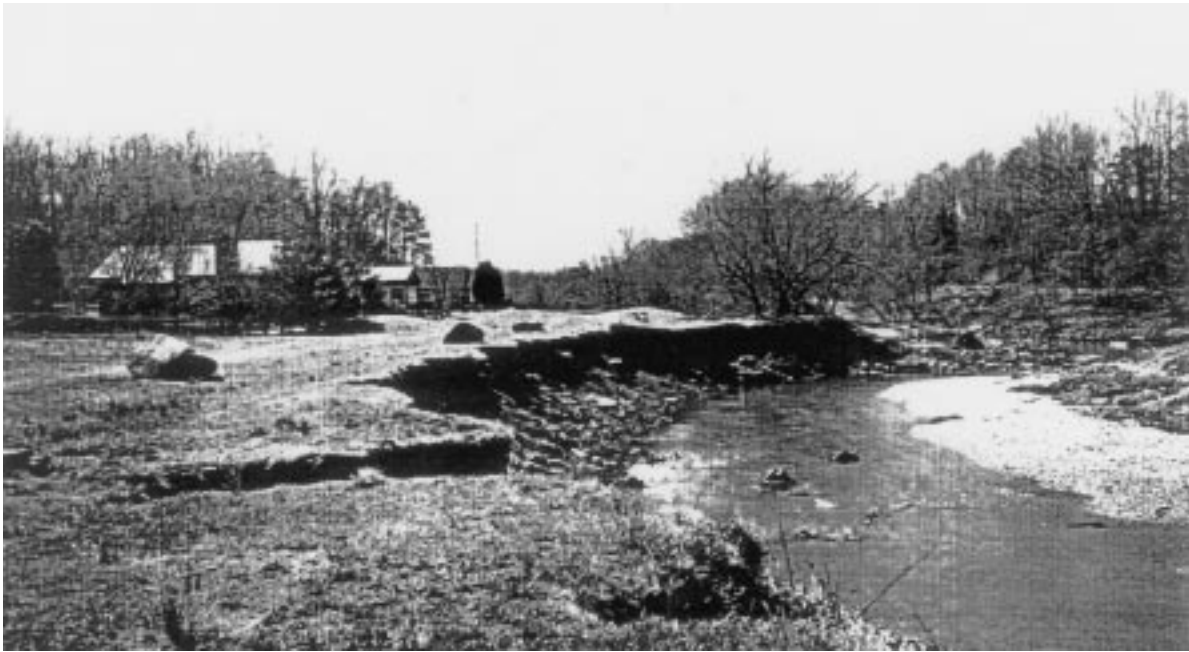
Figure 5. Little Sugar Creek erosion failures before construction.
