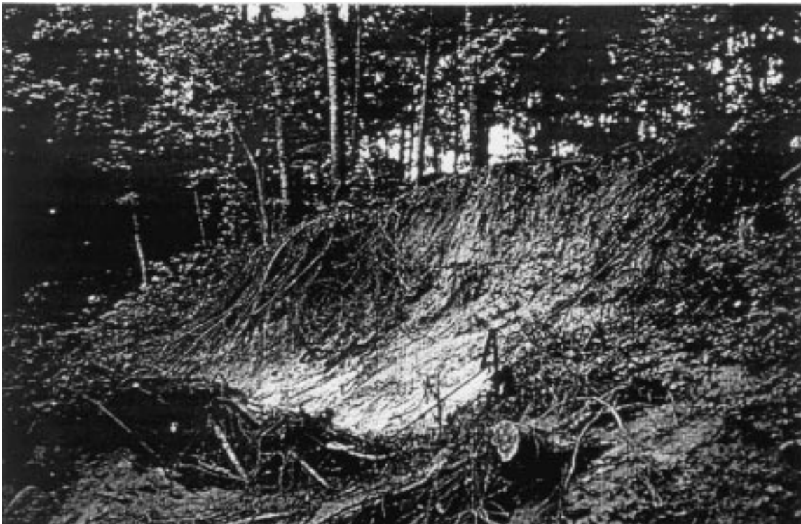
Figure 3. Buffalo Bayou erosional failure after a flood event.
