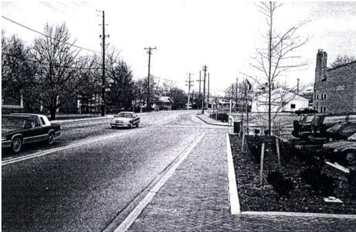
Figure 5. Bioretention streetscaping (planted areas to the right of the street in the photo) help to treat stormwater runoff and improve the appearance of the community.
