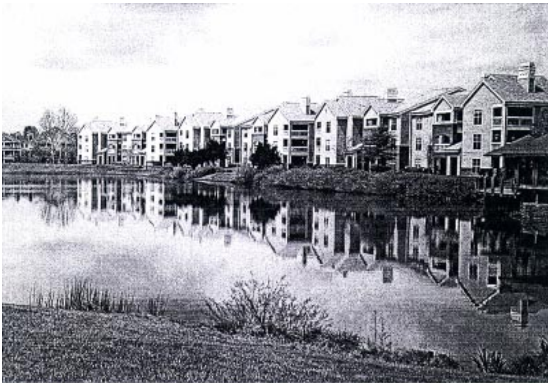
Figure 4. Dry ponds converted to shallow marsh systems improve water quality and enhance the aesthetic beauty of the Port Towns community.
