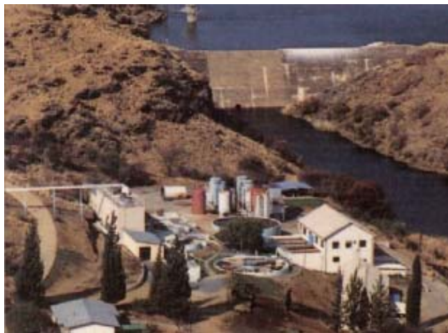
The Goreangab Dam, adjacent to the Windhoek reclamation plant in Windhoek, Namibia. Photo courtesy of Valentina Lazarova
