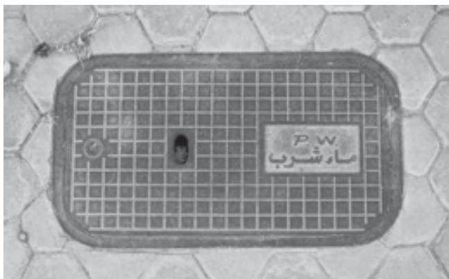
Potable water valve access box on sidewalk on Embassy Row in Riyadh, Saudi Arabia. Photo courtesy of Bahman Sheikh
