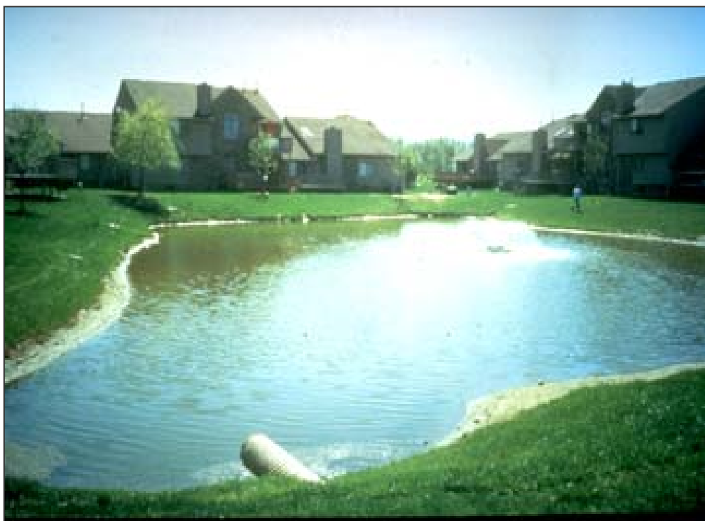
Figure 3 – Example of Wet Pond (courtesy of Hydro Compliance Management, Inc.)
