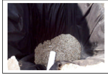
Figures 3, 4. On left, cylindrical infiltration system some 20 feet deep under a subterranean garage for a multi-family building receives roof runoff during a storm and infiltrates into the ground; on right, common box-shaped, sub-surface infiltration trench at a single-family development collects roof and other hardscape runoff for infiltration.
