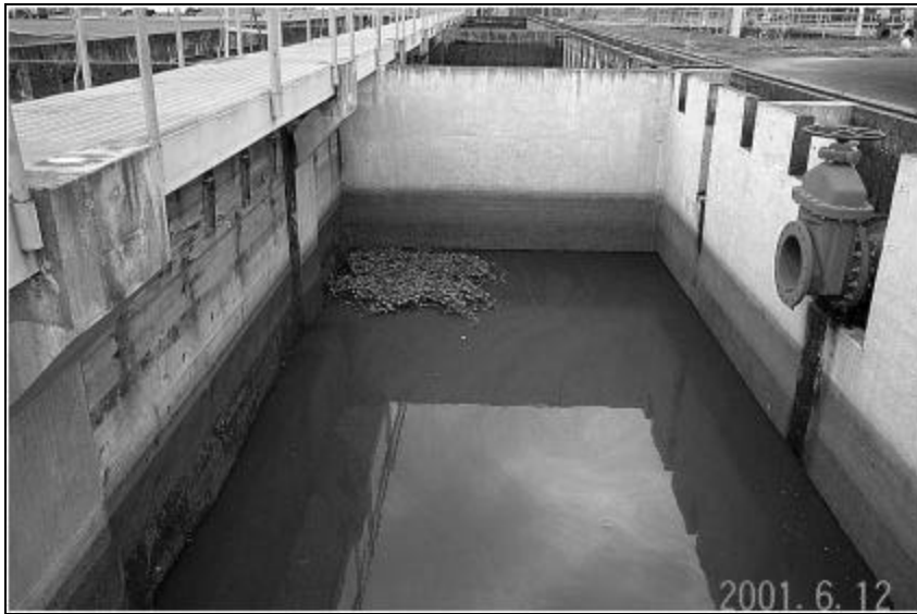
Figure 1 Photograph shows pennywort growing in the first cell of Portland's Vactor© waste decant tank. About three months after its initial introduction into the tank, the pennywort has formed a dense colony about 2.5 m square.
