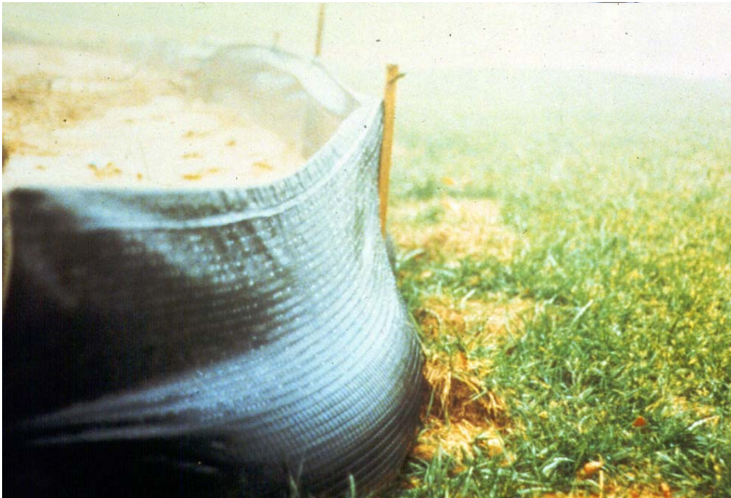
Figure 1 – Example of Silt Fence Containing Sediment -- Geotex ® by SI Geosolutions
