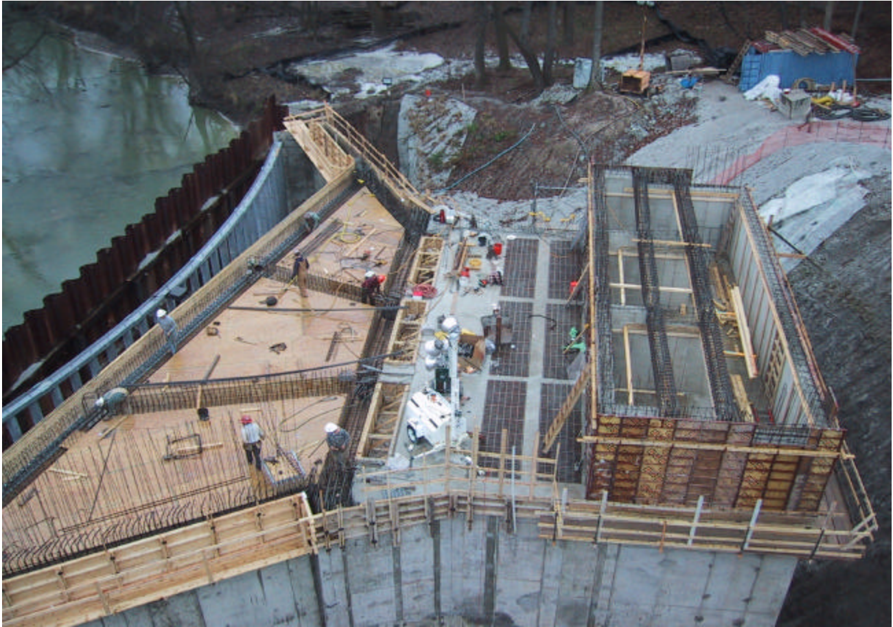
Figure 5. Diversion structure at Thorn Creek during construction
