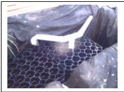
Figures 5, 6. Use of plastic in-fill instead of gravel allows greater storage volume, 94% versus 40%. On left, sub-surface infiltration trench filled with RainStore ; on right, trench filled with StormCell .
