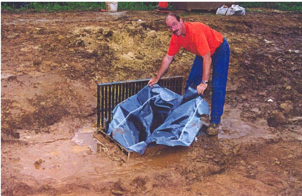
Figure 2 – Example of Type 1 Geotextile Catch Basin Insert -- Siltsack ® by ACF Environmental
