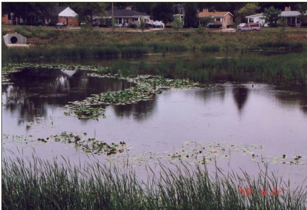
Figure 4 - Example of Constructed Wetland (courtesy of Ingham County, Michigan, Drainage Commission)
