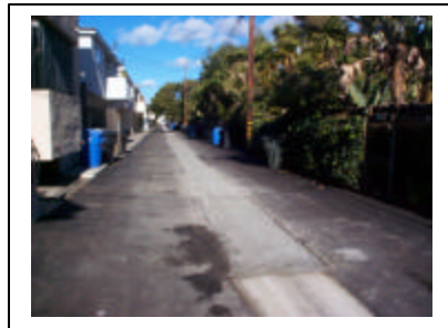
Figure 11. Porous concrete V-swale in a City alley to harvest runoff and reduce flooding of adjacent properties.
