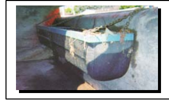
Figures 12, 13. A catch basin insert, DrainPac , captures trash and debris, preventing these materials from entering the receiving waters.
