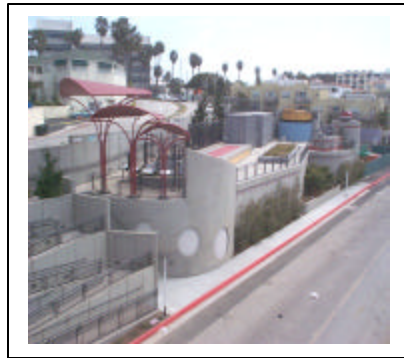
Figure 17. The Santa Monica Urban Runoff Recycling Facility.
