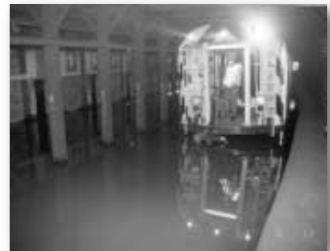
Severe flooding from a water main break compounded the problems in lower Manhattan, forcing a pumping operation that lasted two days and removed 26 million gallons of water from the subway system.
