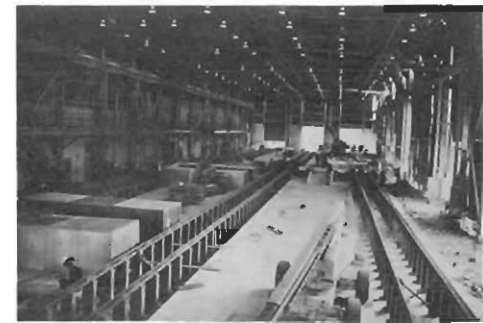
INTERIOR REPAIR SHOP SHOWING FIRST THREE TRACKS
