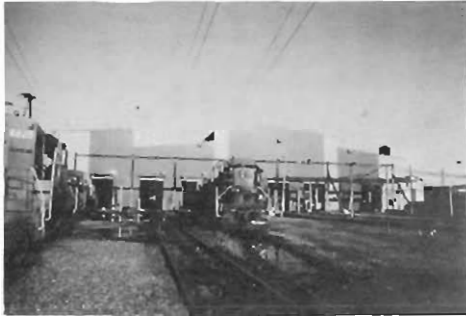
NEW ROOF and SIDING LOCOMOTIVE BUILDING
