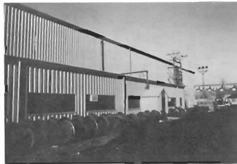
NEW ROOF and SIDING, WHEEL BUILDING
