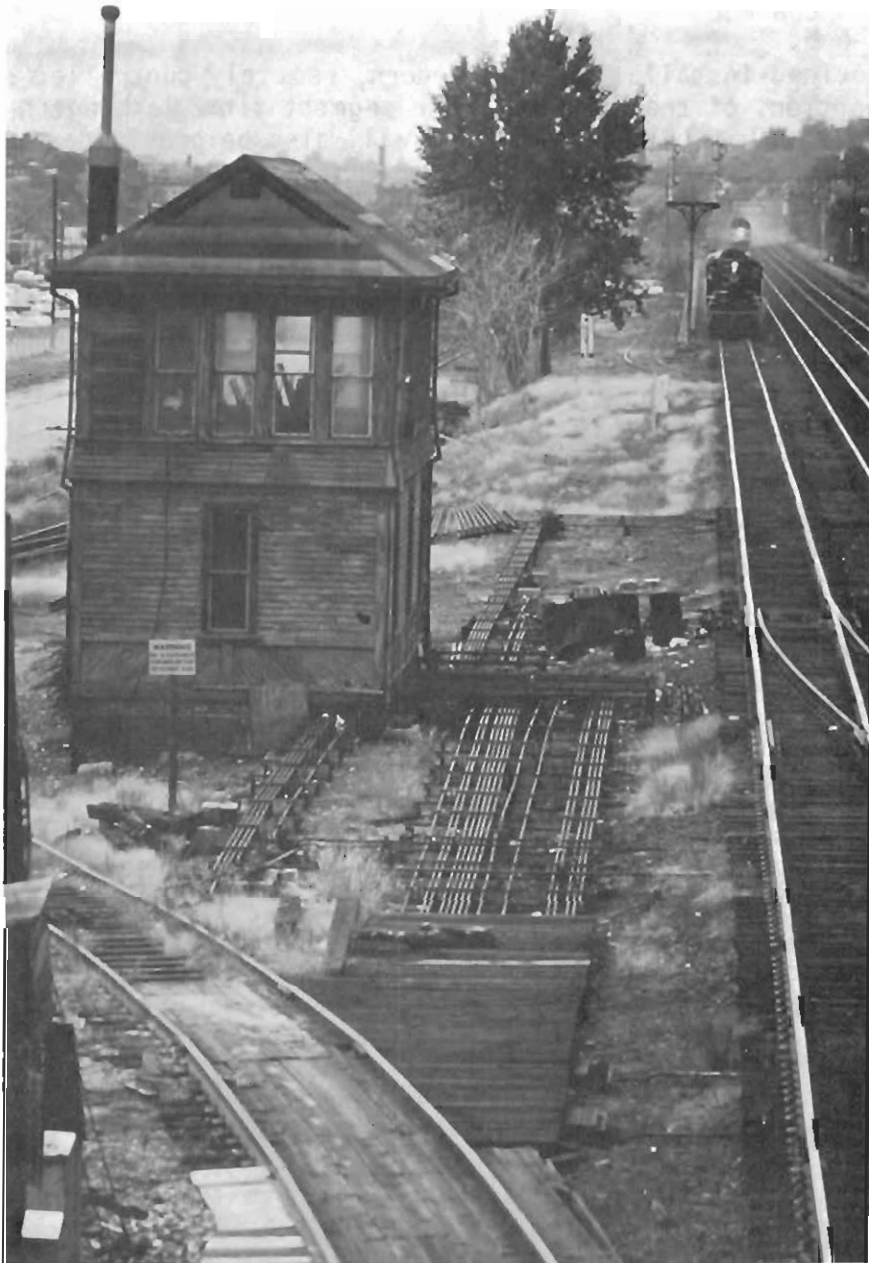
Hand-operated interlocking connected to switches by pipes, vintage 1906. The NECIP converted some, but by no means all, of these antiquated facilities to modern electric operation.
