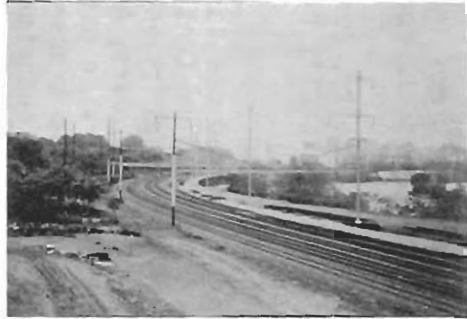
54th STREET and ARSENAL RETAINING WALL
