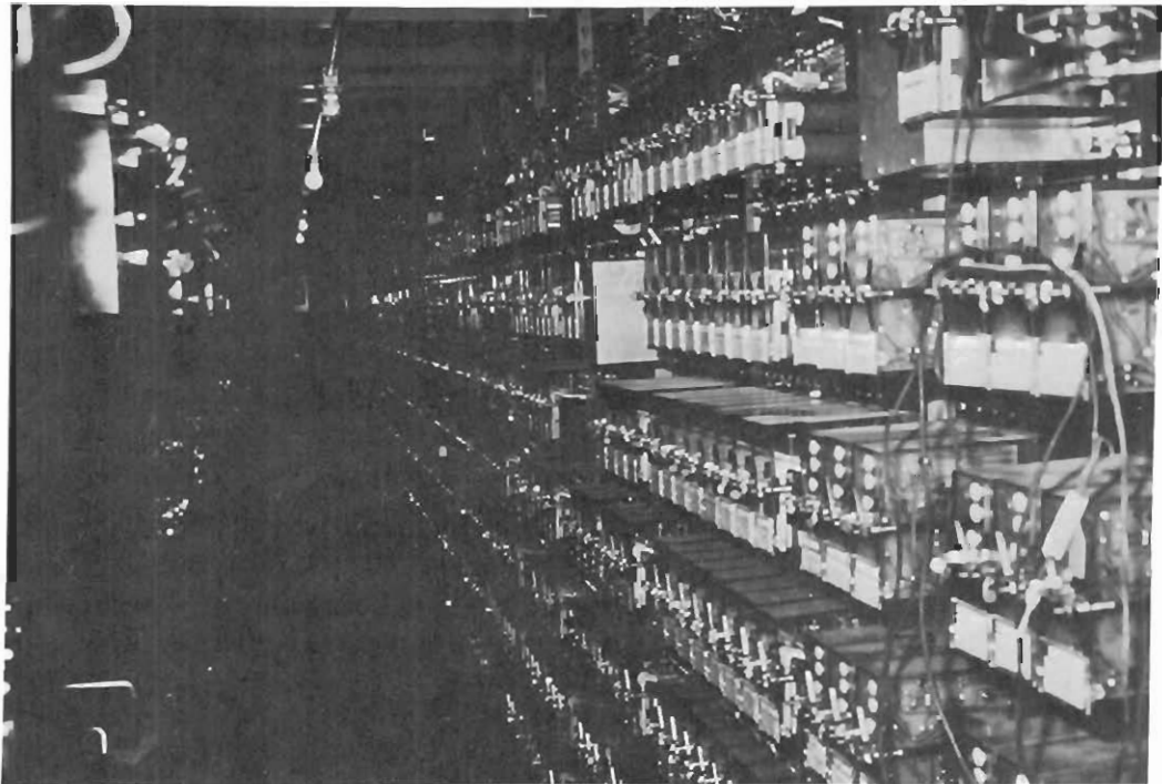
The old and the new: Above, the control levers and lock rods of an old mechanical interlocking (see Chapter 5). Below, the electrical relays controlling a new interlocking built by the NECIP.
