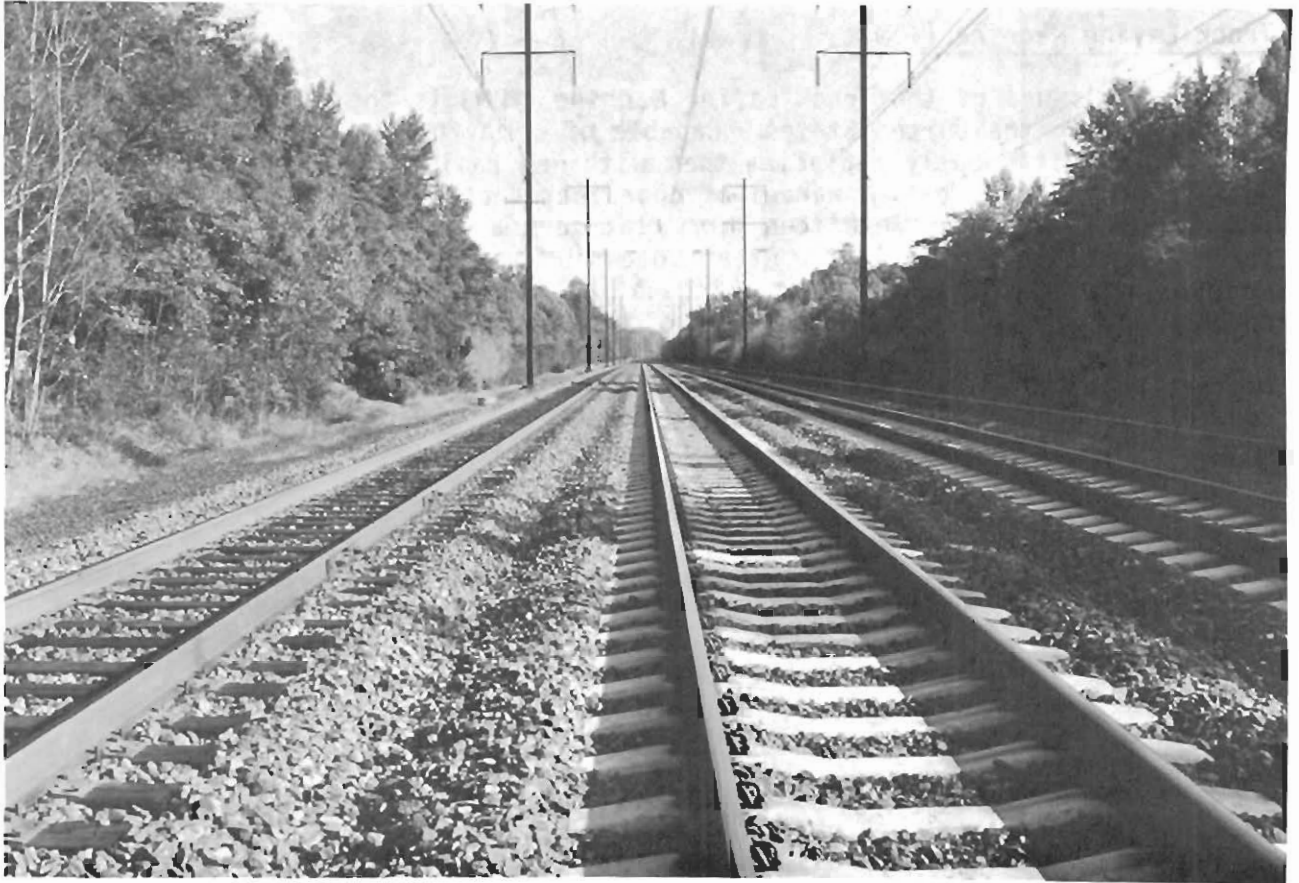
Typical concrete tie installation in multiple-track territory between New York and Washington.
