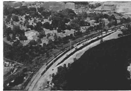
54th STREET and ARSENAL RETAINING WALL
