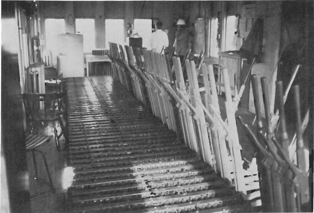
The old and the new: Above, the control levers and lock rods of an old mechanical interlocking (see Chapter 5). Below, the electrical relays controlling a new interlocking built by the NECIP.
