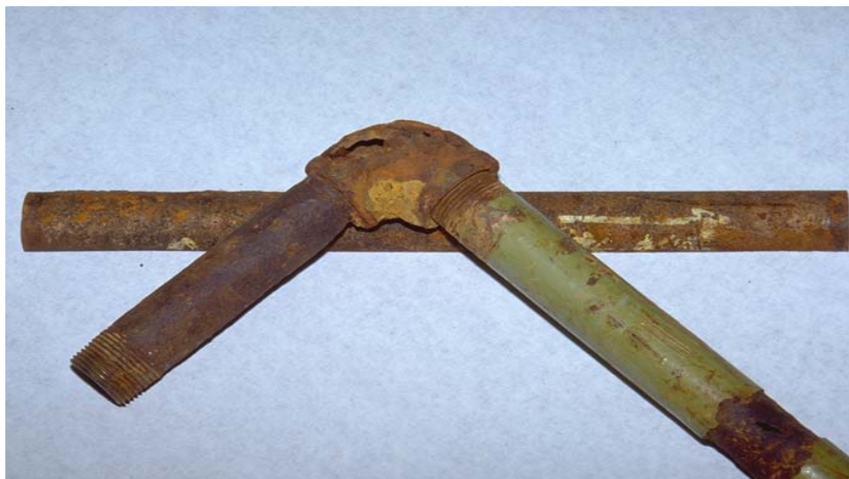
Figure VIII-23 Poor Construction Practice
