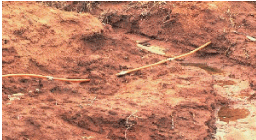
Example of a washout area found by patrol.
