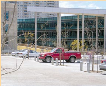
left: A VEGETATED SWALE FILTERS WATER TO HELP RESTORE THE PREDEVELOPMENT HYDROLOGY OF THE SITE AT THE SSA TELESERVICE CENTER IN AUBURN, WASHINGTON.
