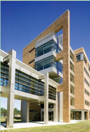
above: THE FDA CAMPUS IN WHITE OAK, MARYLAND, USES A COGENERATION PLANT FOR ELECTRICITY, HOT WATER, AND STEAM.
