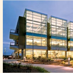
NATIONAL PARK SERVICE MIDWEST REGIONAL HEADQUARTERS OMAHA, NE
