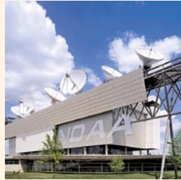
NOAA SATELLITE OPERATIONS FACILITY SUITLAND, MD LEED NC rated: Oct 26 2007
