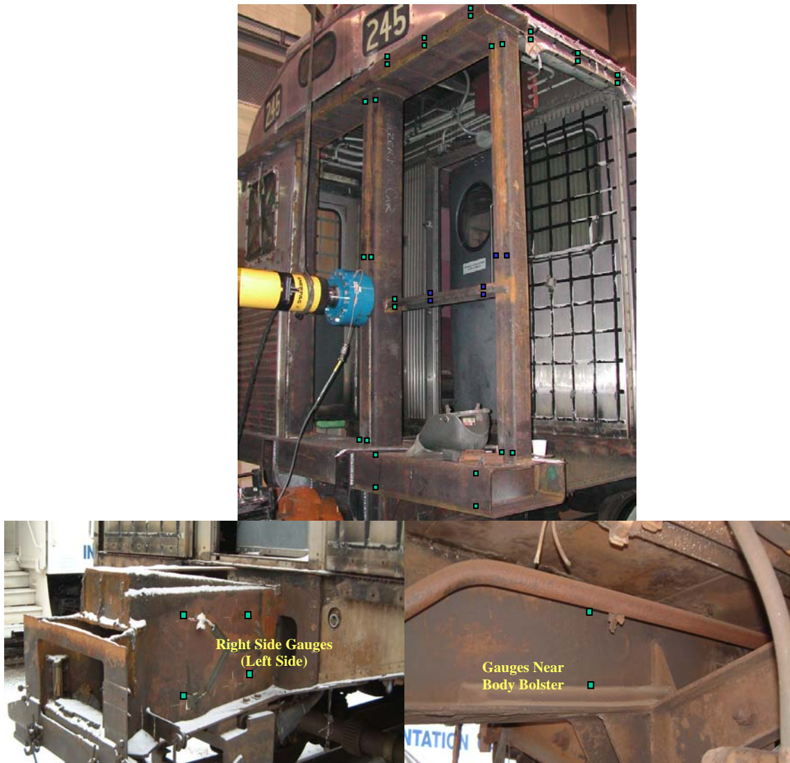
Figure A-6. Gauge Locations at the End Structure and Under Structure of a 1990s Design Carbody
