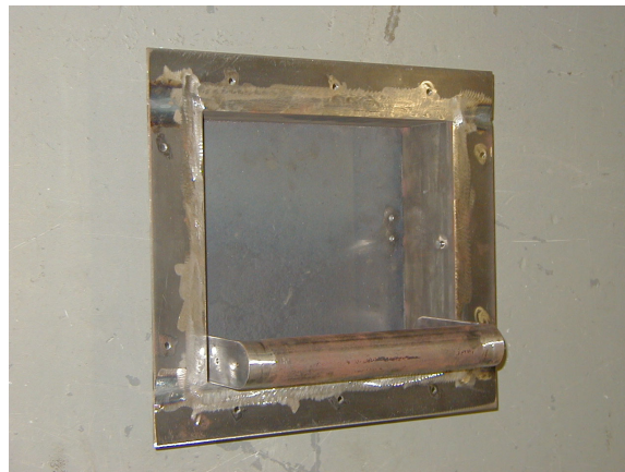
Figure 21. Hand/fothold in the deployed condition
