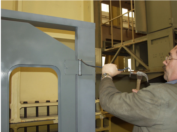
Figure 79. Removal of the pin-insert from the hinge pin
