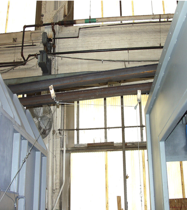
Figure 29. Pulleys remove hatch from egress path
