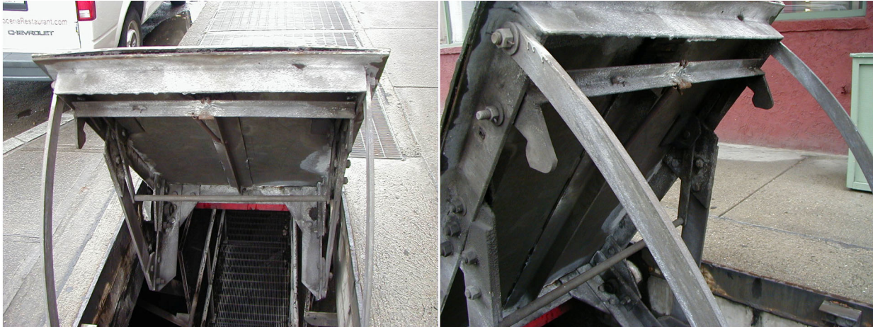
Figure 15. Sidewalk Hatch for Subway System, Boston, MA
