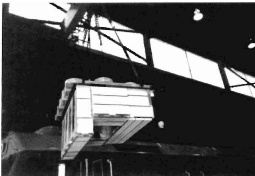
Figure 78. The Cool Box Being Raised for Installation in the Locomotive
