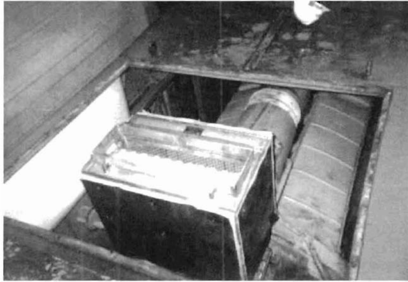
Figure 76. The New APECS Exhaust Silencer Installed on the Ernest Marsh
