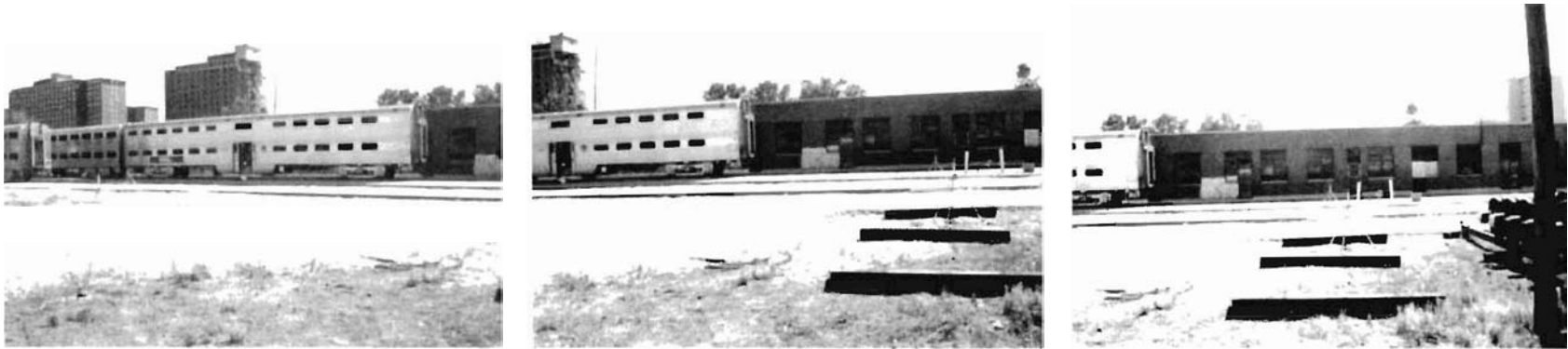
Figure 83. The Test Site at the Chicago Metra 51st St. Yard
