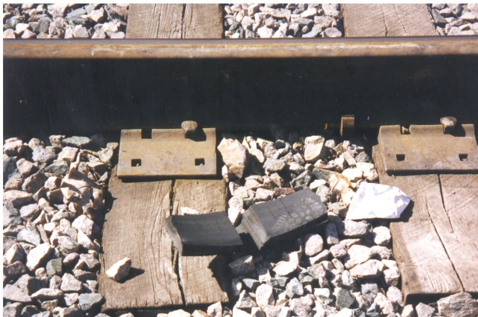
Figure 3. Example of debris on the ground of a railroad yard
