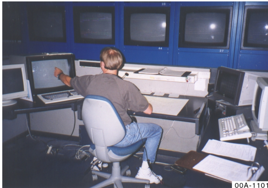
Figure C-1. Dispatching desk at pilot site No. 1
