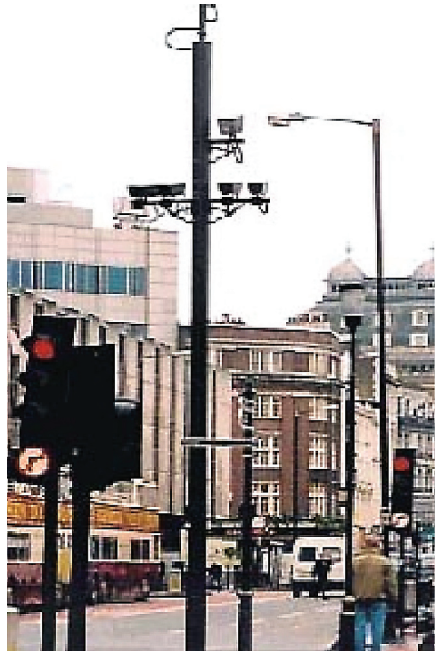
Enforcement cameras in London are installed on existing utility poles
