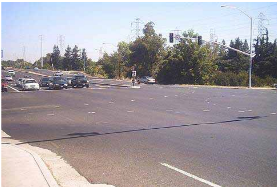
Figure 21. Picture of Howe Avenue and College Town Drive Intersection
