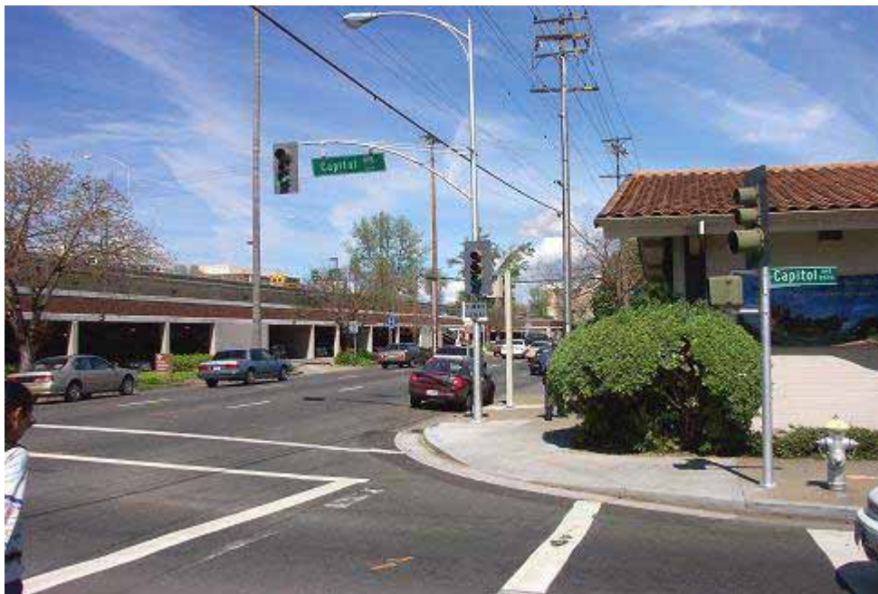
Figure 17. Picture of 30 th Street and Capitol Avenue Intersection
