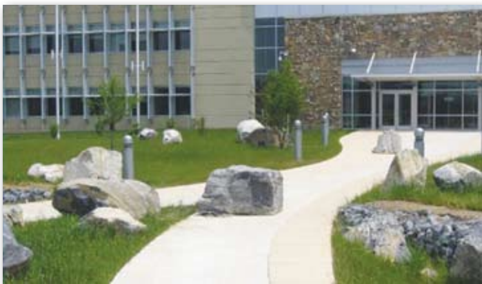
Boulders excavated from the construction site were reused as natural security bollards.
