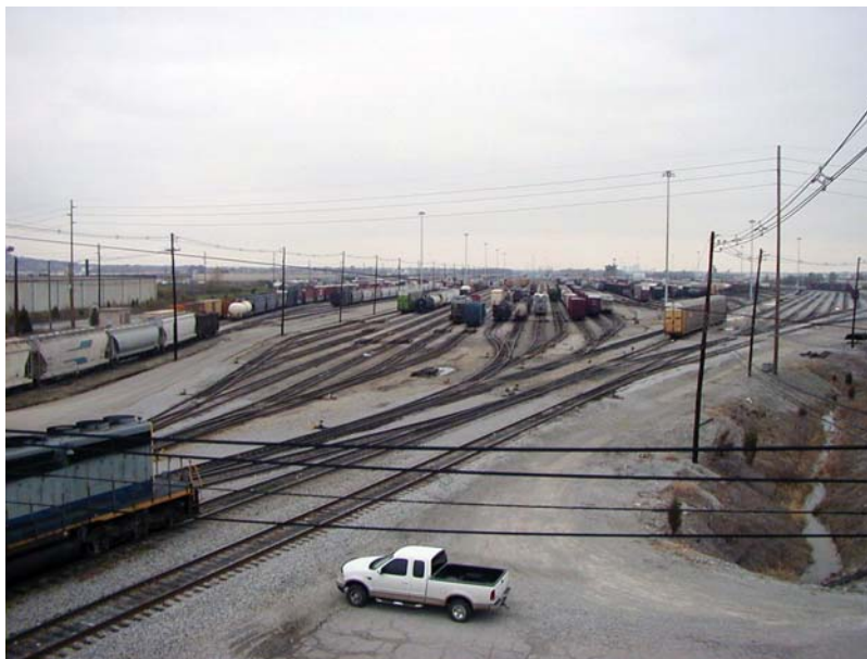
Figure 1. Railroad classification (switching) yard
