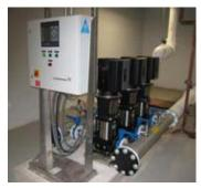
GSA recently replaced the domestic water pumping station at the RAY Building. The original pumping station was installed during the building renovation in 1987-1990. It was a constant speed motor system that used regulators and a combination of pumps to maintain water pressure to the building above the third floor. The system's water pressure varied over a wide range and the pumping station required frequent repairs.
