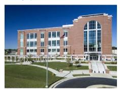
The courthouse is situated on a three-acre site and rests on 170 concrete piers, which are socketed into solid bedrock at depths up to 65 feet; making the building able to withstand significant seismic events.
