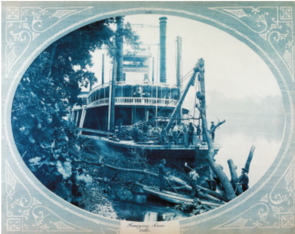
Figure 3-4. Snag clearing in 1885 (top photo) contributed to the instability of the river bank because trees were removed 100 to 200 feet (30 to 60 m) back from the shoreline to reduce future hazards. Wing dams constructed in 1891 by placing consecutive layers of willow mats and rock together (bottom photo) were used to constrain the channel, increase water levels, scour the channel, and reduce shoreline erosion (Source: John Anfinson, U.S. Army Corps of Engineers, St. Paul District, St. Paul, Minnesota).
